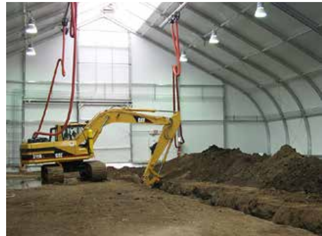
A temporary enclosure system is one method to extend construction activity into winter season.
