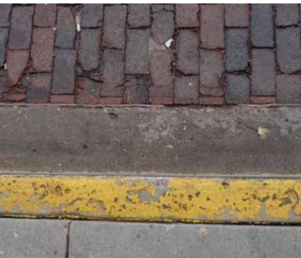
Deteriorated brick paving
