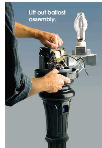
REMOVING BALLAST ASSEMBLY
