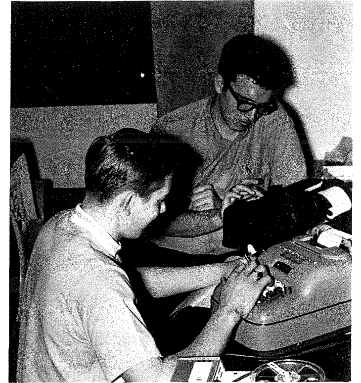
Randy Buck and Gordon Longden work on totals.
