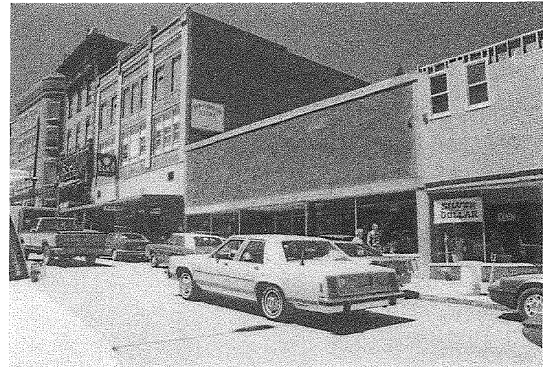
Earlier infill buildings on Main Street
