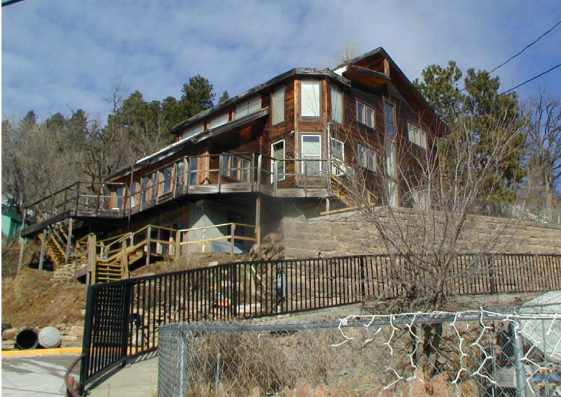
The building was not built during the period of historic significance. Fenestration patterns and overall design are not historic.
