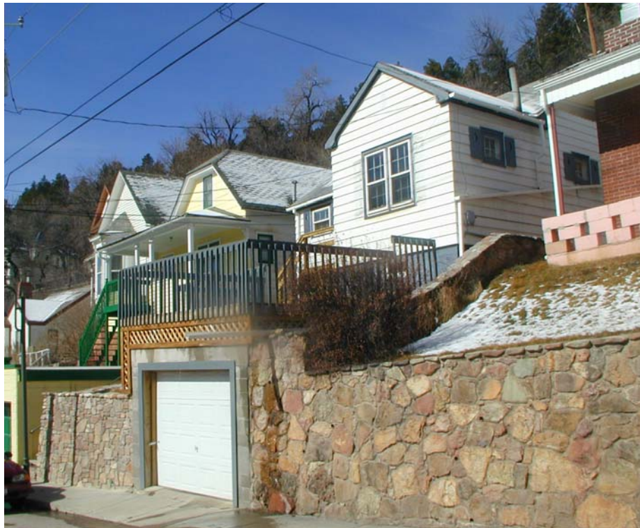
Deck railings are an important design consideration.
