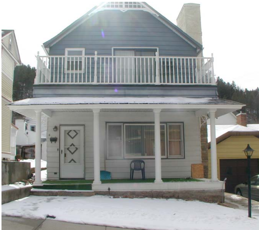
First floor porch restoration used columns appropriate in style and material. Second floor railing is well designed.
