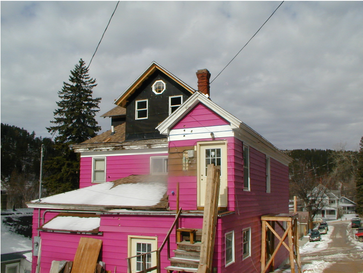
This dormer addition is on the rear of the house. The roof line of the dormer mimics the historic roof lines. The dormer is appropriately sized for the house and does not disturb the existing volumes.
