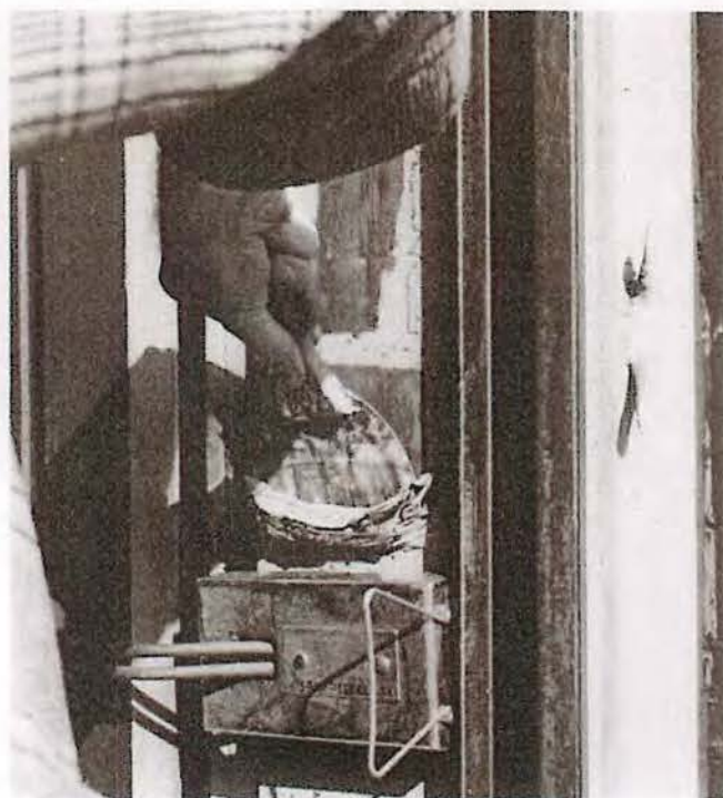
Fig. 13 The electric heat plate (with paint scraper) is particularly useful for removing paint down to bare wood on flat surfaces such as doors, window frames, and siding. After scraping, some light sanding will probably be necessary to smooth the surface prior to application of primer and top coats. Photo: David W. Look, AIA.
