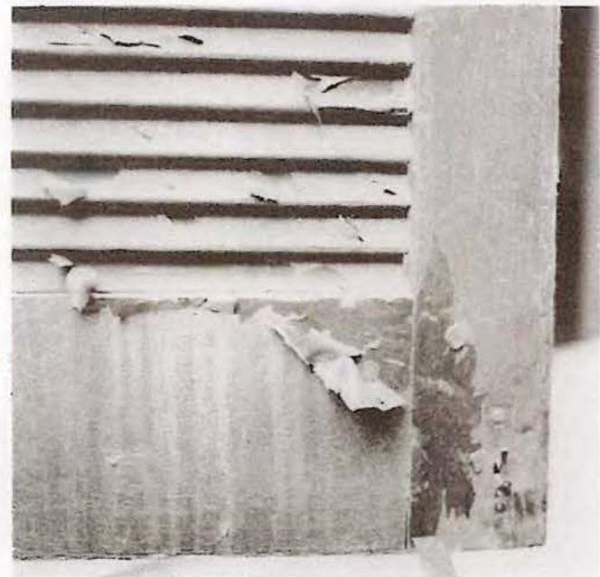
Fig. 6 This is an example of intercoat peeling. A latex top coat was applied directly over old oil paint and, as a result, the latex paint was unable to adhere. If latex is being used over oil, an oil-base primer should be applied first. Although much of the peeling latex paint can be scraped off, in this case, the best solution may be to chemically dip strip the entire shutter to remove all of the paint down to bare wood, rinse thoroughly, then repaint. Photo: Mary L. Oehrlein, AIA.
