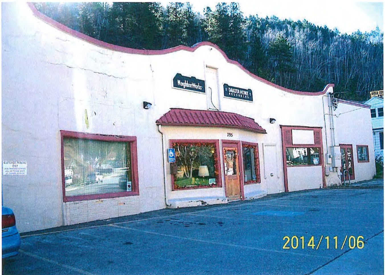
Front of Building
