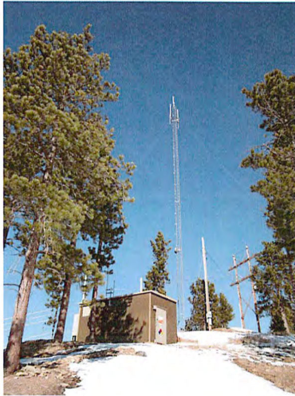
20861 Spruce Gulch Rd. Existing Tower
