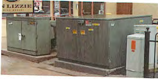
Current look of Utility Box
