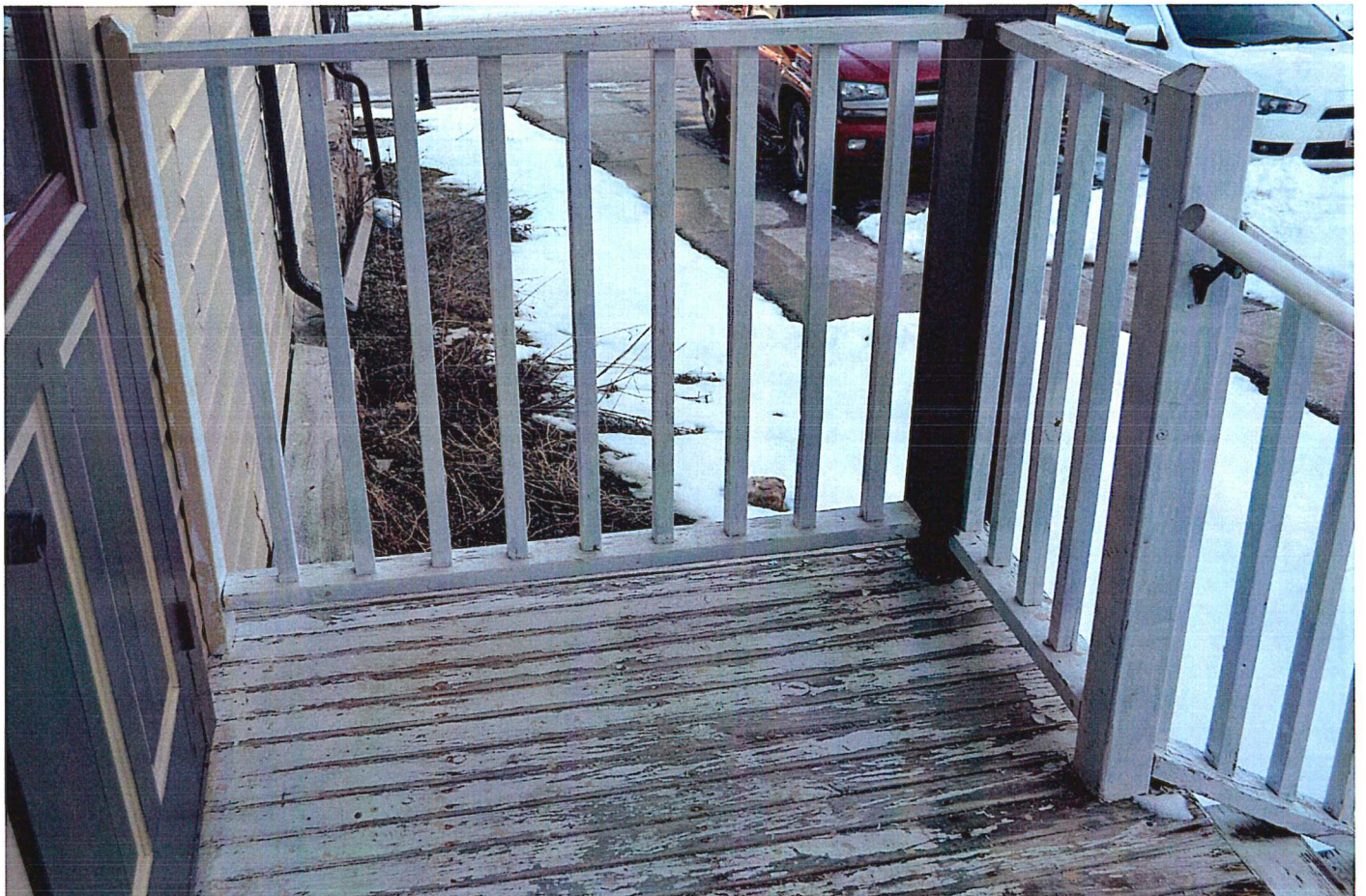
Other side of 2nd porch has some soft places in the wood floor & rails are weak
