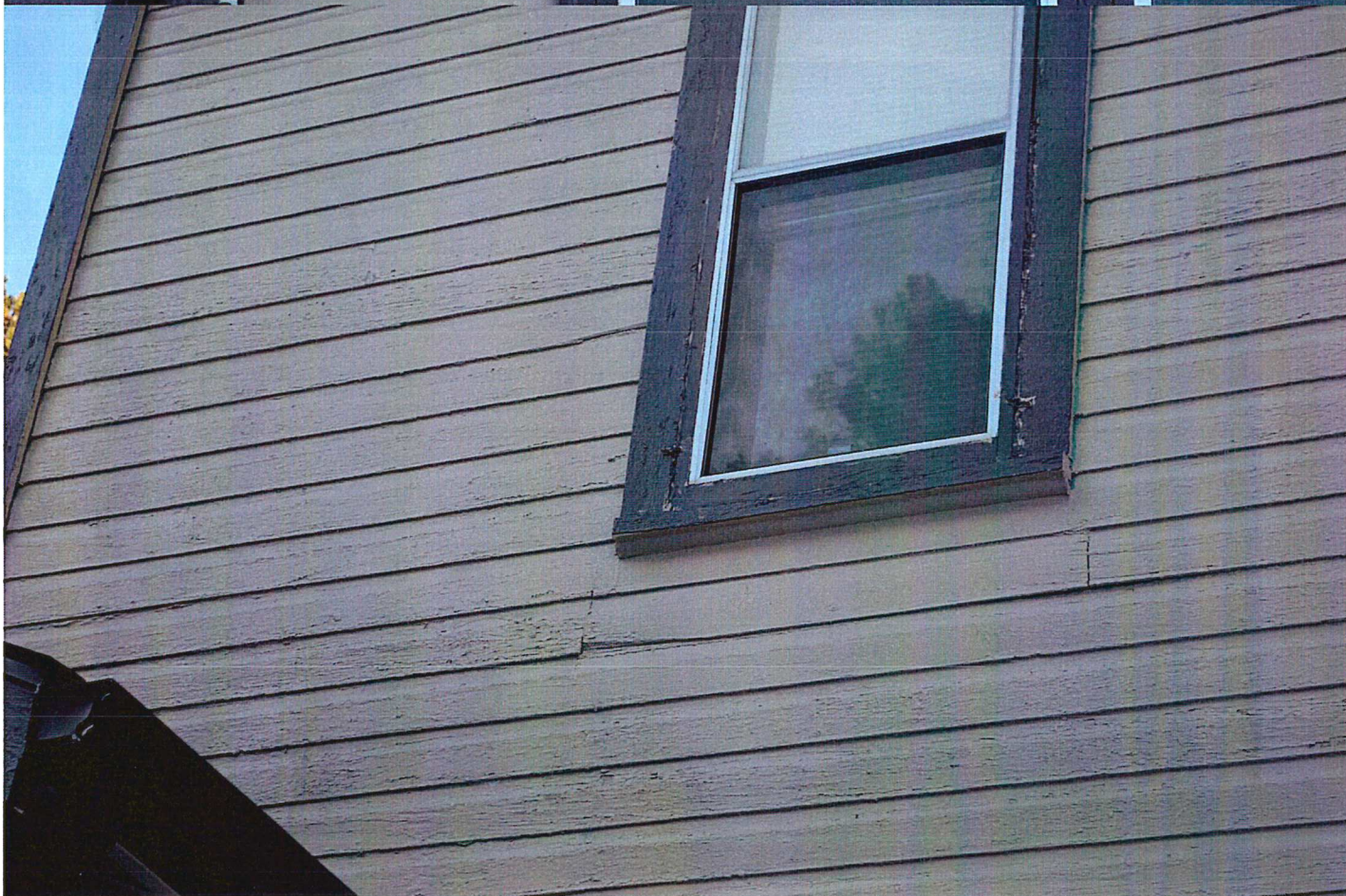
Lower window wood cracking
