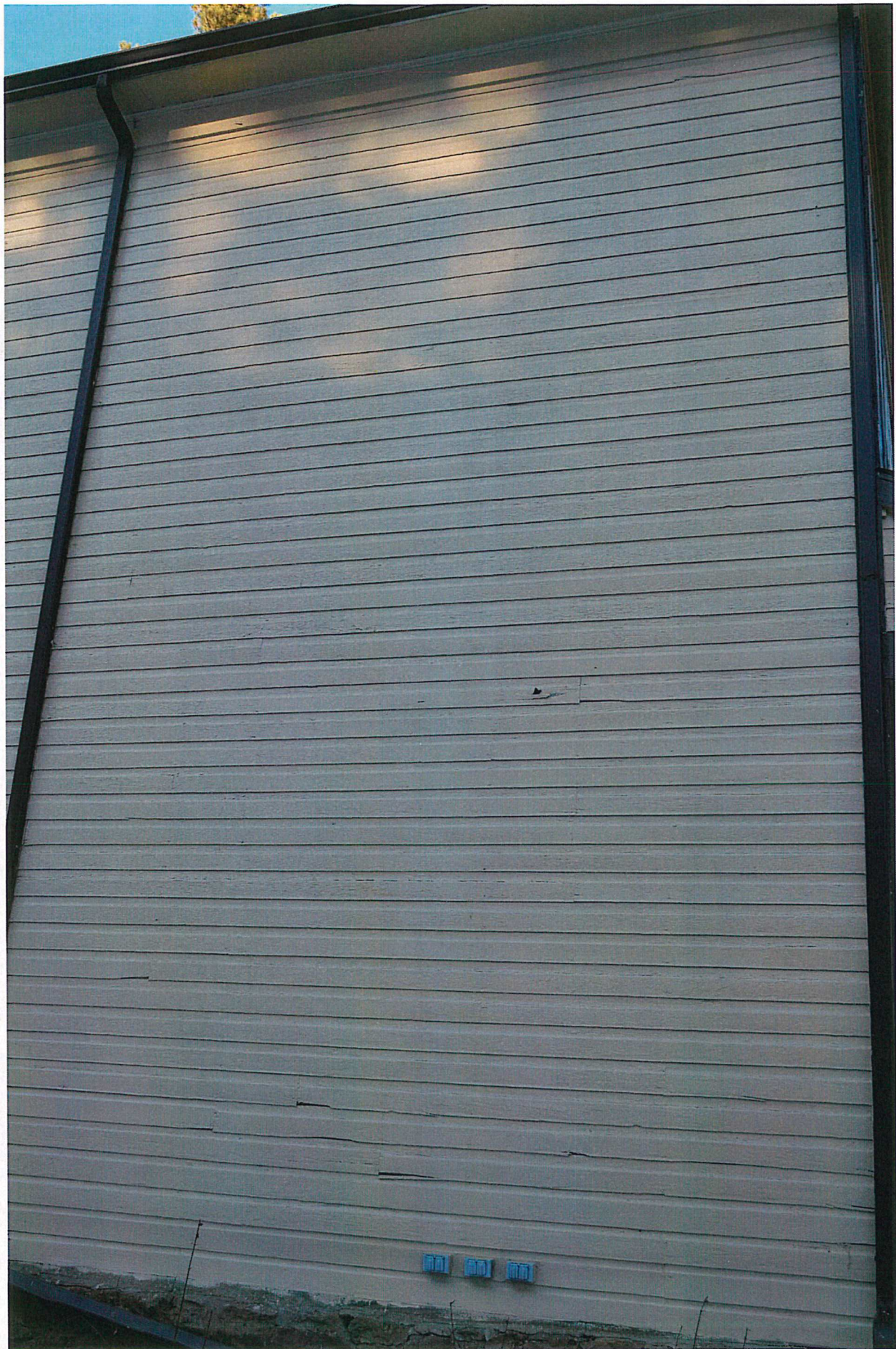
158 Williams St. South Facing Wall, Hard to see all cracks but they are everywhere, top to bottom + Broken out pieces
