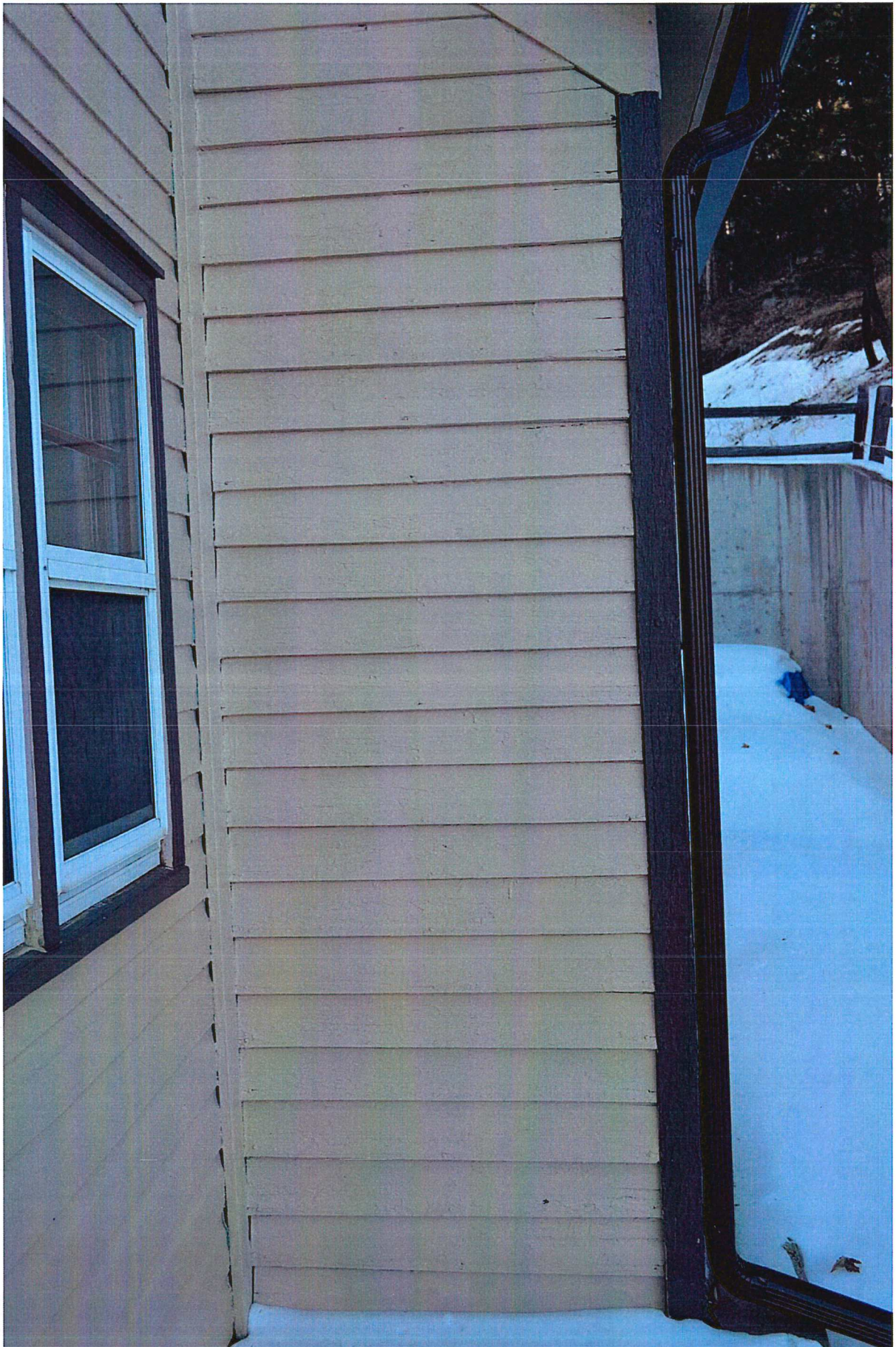
East facing short wall has lots of cracks along edges & siding don't match original wood siding
