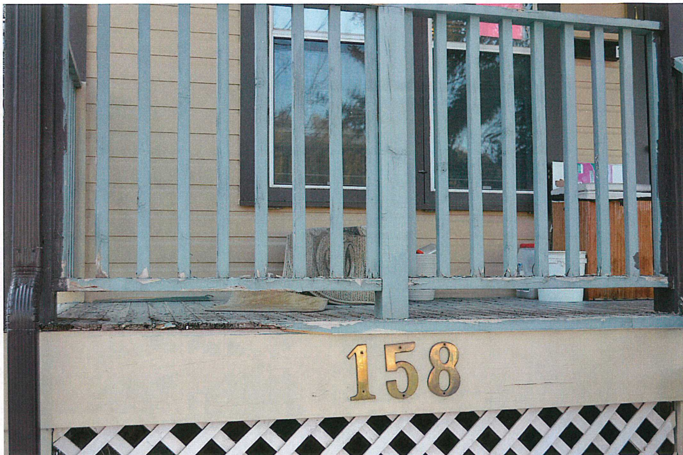
Wood decking is rotting out in Corner Area
