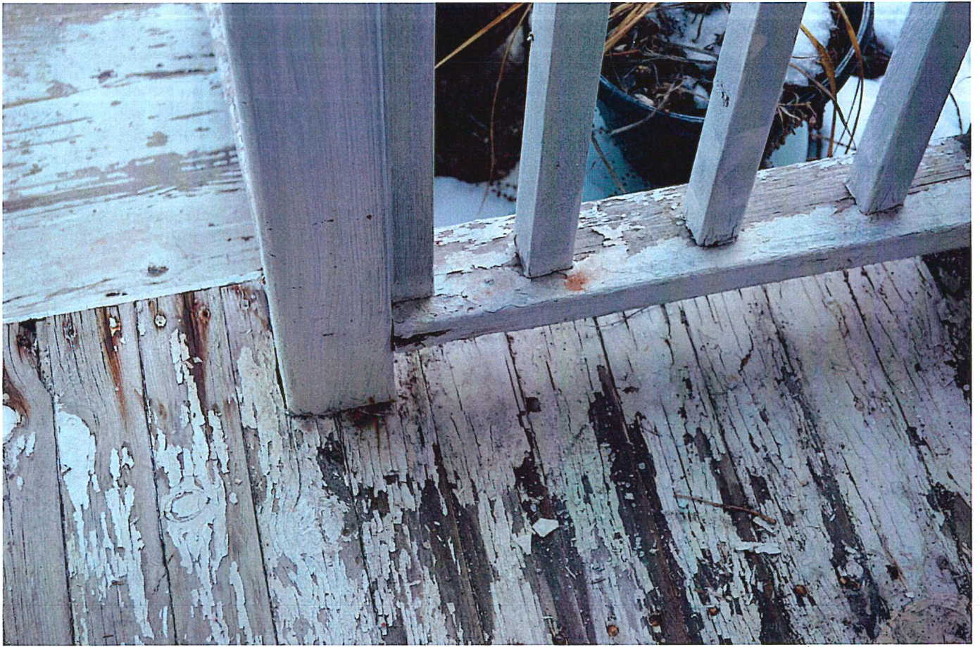
Most railing is cracked & weakened
