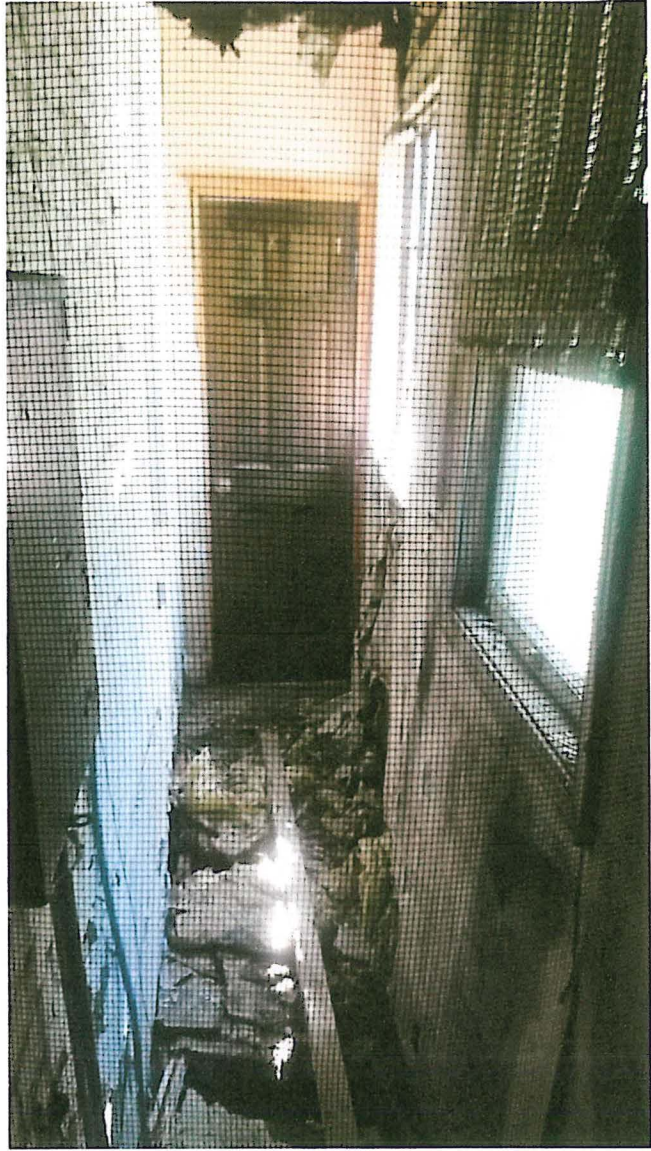
Rotted and collapsing porch addition – removed 2015
