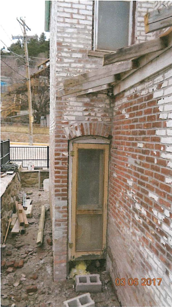
Original back entry with masonry stabilized
