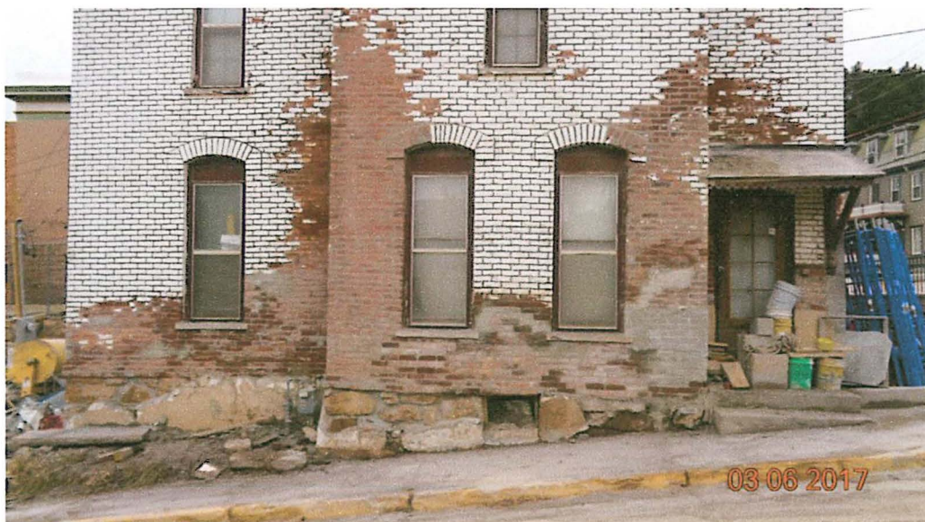
Masonry veneer stabilization in process
