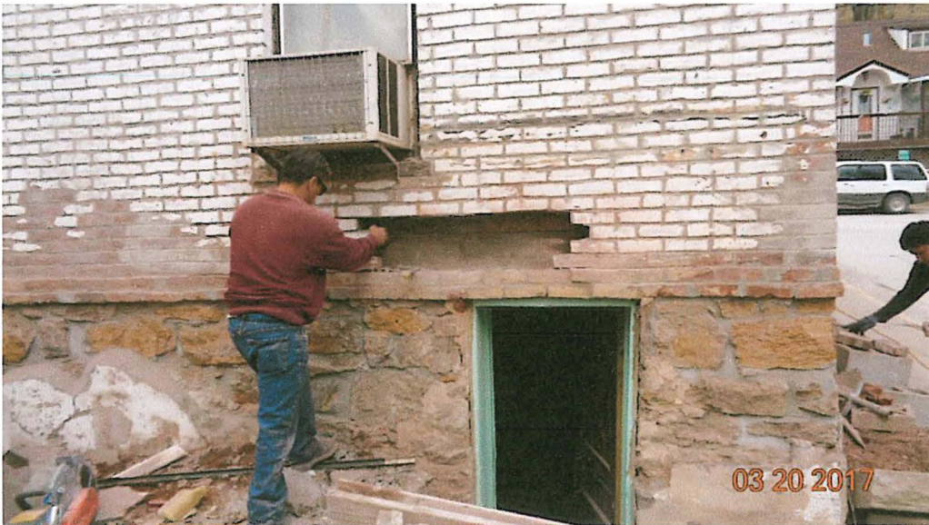
Phase II – inserting cavity flashing system
