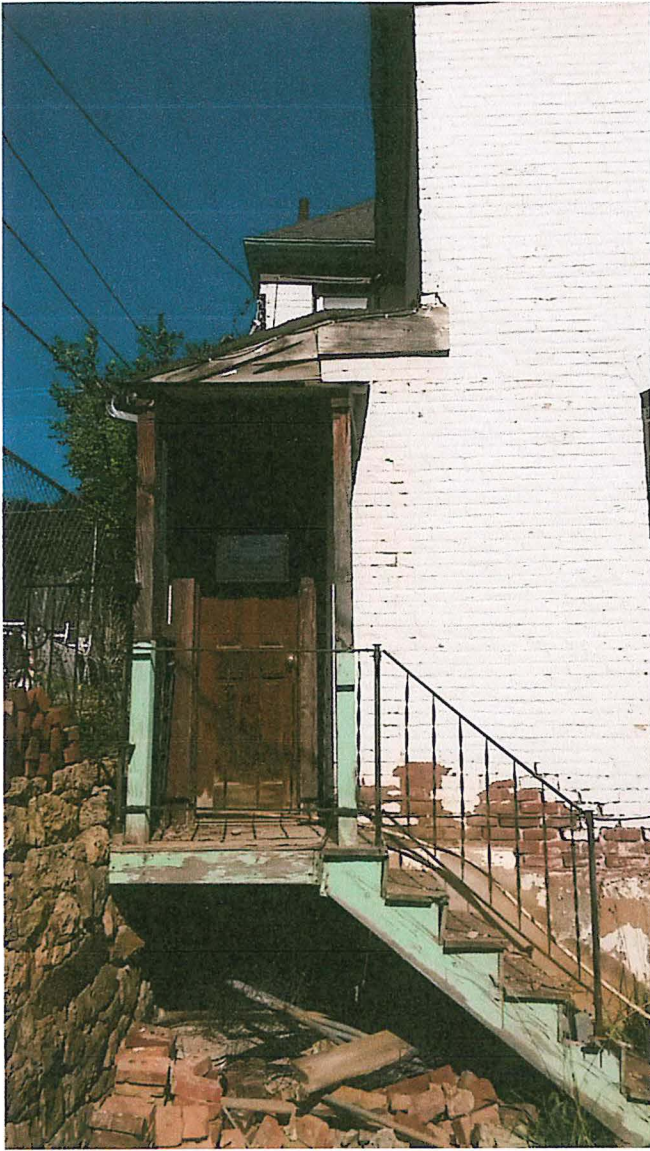
Rotted and collapsing porch addition – removed 2015
