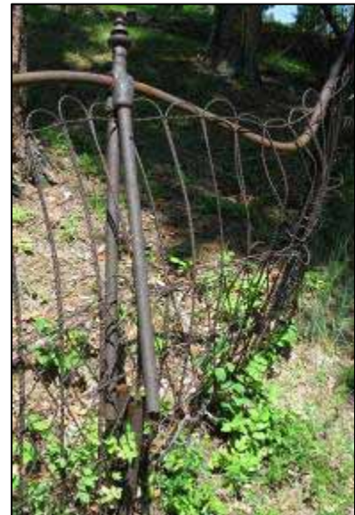
Example of ironwork damaged from falling tree limb.
