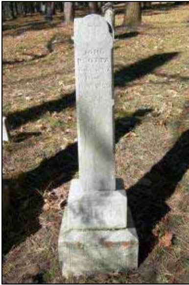
The John Psotta monument as photographed in November, 2007. Biological growth has not returned in the 4 years since cleaning.
