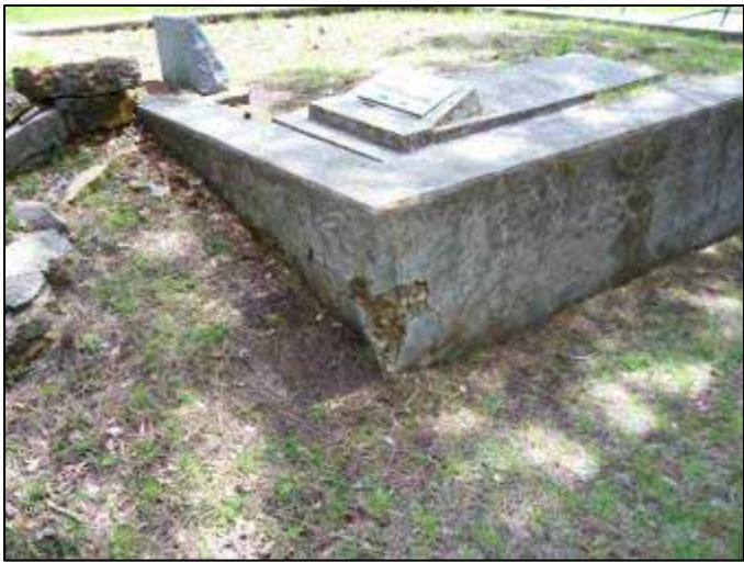
Photo 3.3 - Surface Spalling
