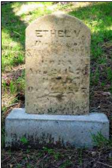
This small sandstone monument is a high priority candidate for stone consolidation. Much of the gravestone data has been lost but what remains is in dire need of conservation.
