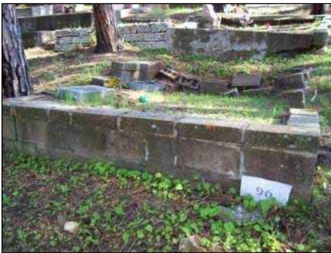
Photo 3.10 – Masonry Wall with Different Levels of Repair
