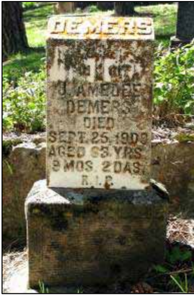
The marble headstone and limestone base at the Demers gravesite would be a good candidate for cleaning.
