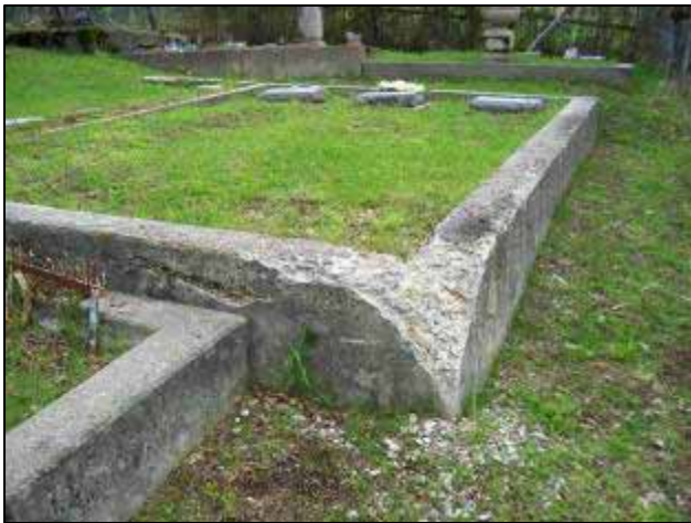
Photo 3.2 - Freeze-Thaw Deterioration
