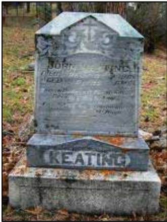
Figure 2.3 – A Low Priority gray marble monument with a limestone base in a stable condition.
