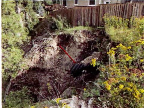
Figure 2 – Erosion below the cul-de-sac and pipe protruding from the bank.
